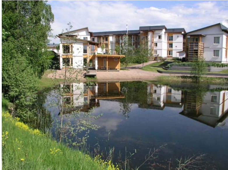
Experimental area for timber construction
