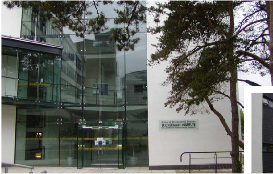
Left and below: The ZICER building emphasised low energy consumption from the start.
